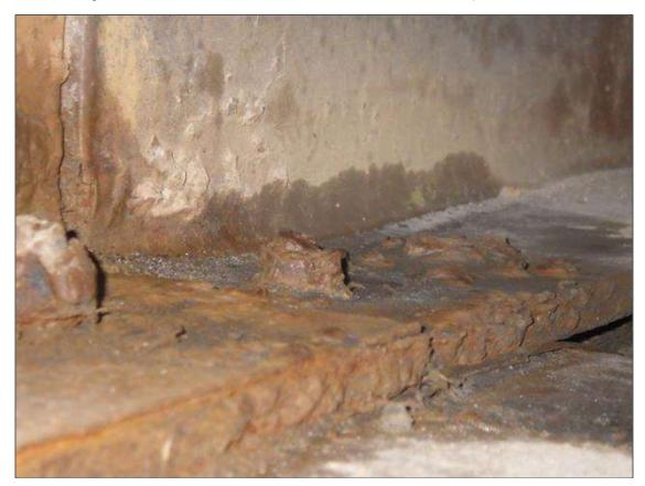
Span 1 Near Bearing: MISSING LEFT ANCHOR BOLT NUT IN BEAM 3 BEARING (PRIORITY ACTION REQUEST)
