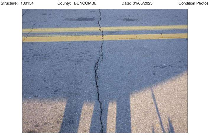
Span 2 Wearing Surface: TRANSVERSE CRACK UP TO FULL WIDTH X 1/4 INCH WIDE AT END BENT 2
