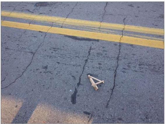
Span 2 Wearing Surface: TRANSVERSE CRACKS UP TO FULL WIDTH X 1/8 INCH WIDE AT LESS THAN 1 FOOT SPACING ALONG THE DECK BOARD EDGES THROUGHOUT
