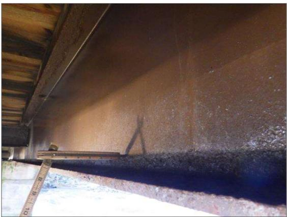
Span 2 Beam 2: ARRESTED CORROSION UP TO INTERMITTENT FULL LENGTH X 8 INCHES HIGH WITH 1/32 INCH SECTION LOSS IN THE WEB
