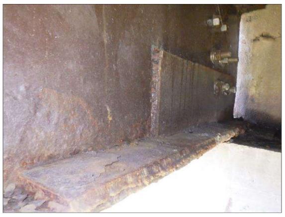
Span 1 Beam 9: (4) REPAIR PLATES (1) UP TO 3 FEET LONG X 3 1/2 INCHES WIDE X 1/2 INCH THICK IN THE LEFT BOTTOM FLANGE, (2) UP TO 2 FEET LONG X 7 INCHES HIGH X 3/4 INCH THICK IN THE LEFT AND RIGHT SIDES OF THE WEB, AND (1) UP TO 4 FEET LONG X 3 1/2 INCHES WIDE X 1/2 INCH THICK IN THE RIGHT BOTTOM FLANGE AT END BENT 1 Structure: 10154 County: BUNCOMBE Date: 01/05/2023 Condition Photos
