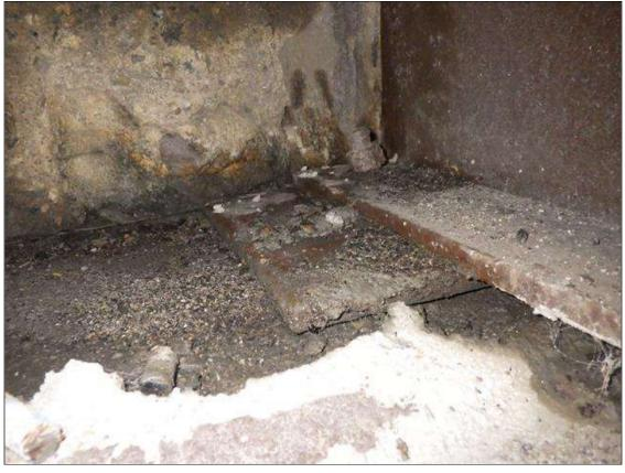
BEAM 8 BEARING AT END BENT 2 REPAINTED PRIOR TO 2023 INSPECTION CYCLE (OTHERS SIMILAR, OTHERS AT END BENT 1 SIMILAR)
