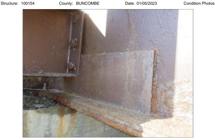
Span 1 Beam 9: (4) REPAIR PLATES (1) UP TO 3 FEET LONG X 3 1/2 INCHES WIDE X 1/2 INCH THICK IN THE LEFT BOTTOM FLANGE, (2) UP TO 2 FEET LONG X 7 INCHES HIGH X 3/4 INCH THICK IN THE LEFT AND RIGHT SIDES OF THE WEB, AND (1) UP TO 4 FEET LONG X 3 1/2 INCHES WIDE X 1/2 INCH THICK IN THE RIGHT BOTTOM FLANGE AT END BENT 1
