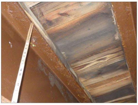
Span 2 Beam 6: ARRESTED CORROSION UP TO INTERMITTENT FULL LENGTH X FULL WIDTH WITH 7/16 INCH REMAINING (GREATER THAN OR EQUAL TO 1/16 INCH SECTION LOSS, LESS THAN 25 PERCENT SECTION LOSS) IN THE TOP FLANGE
