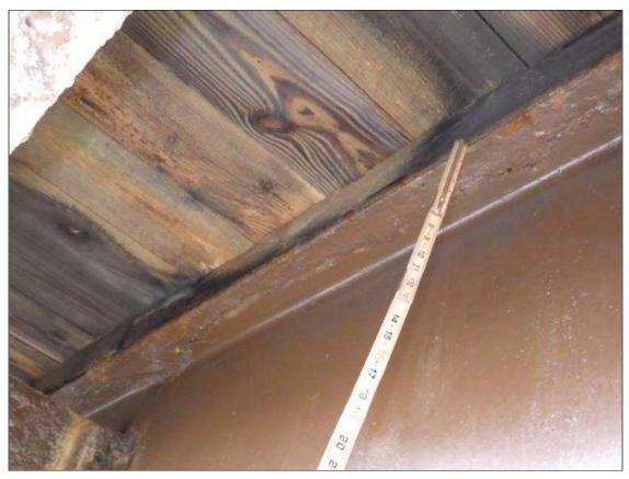
Span 1 Beam 6: ARRESTED CORROSION UP TO FULL LENGTH X FULL WIDTH WITH 7/16 INCH REMAINING (GREATER THAN OR EQUAL TO 1/16 INCH SECTION LOSS, LESS THAN 25 PERCENT SECTION LOSS) IN THE TOP FLANGE
