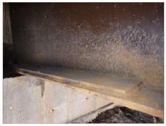
Span 1 Beam 7: (2) REPAIR PLATES UP TO 2 FEET 6 INCHES LONG X 3 1/2 INCHES WIDE X 1/2 INCH THICK IN THE BOTTOM LEFT FLANGE AND 3 FEET 4 INCHES LONG X 3 1/2 INCHES WIDE X 1/2 INCH THICK IN THE BOTTOM RIGHT FLANGE AT END BENT 1
