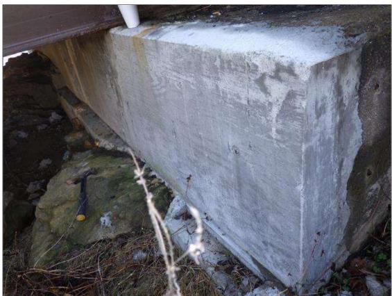
End Bent 1 Abutment: REPAIR PATCH AREA UP TO FULL LENGTH X 3 FEET HIGH X 7 INCHES THICK
