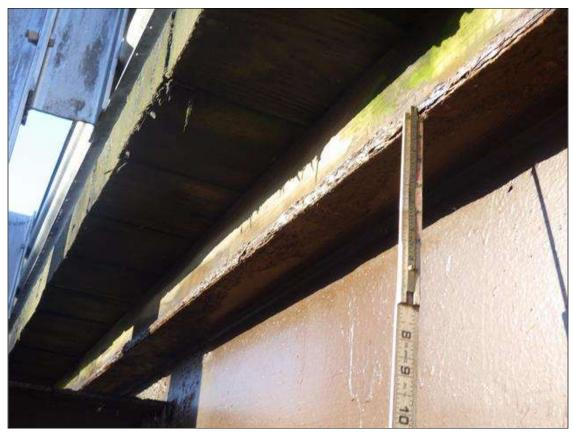
Span 2 Beam 9: ARRESTED CORROSION UP TO INTERMITTENT FULL LENGTH X FULL WIDTH WITH 3/8 INCH REMAINING (GREATER THAN OR EQUAL TO 1/16 INCH SECTION LOSS, GREATER THAN 25 PERCENT SECTION LOSS) IN THE TOP FLANGE (PRIORITY ACTION REQUEST)
