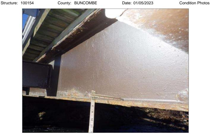
Span 1 Beam 9: ARRESTED CORROSION UP TO INTERMITTENT FULL LENGTH X 5 INCHES HIGH WITH 5/16 INCH REMAINING (GREATER THAN OR EQUAL TO 1/16 INCH SECTION LOSS, LESS THAN 25 PERCENT SECTION LOSS) IN THE WEB
