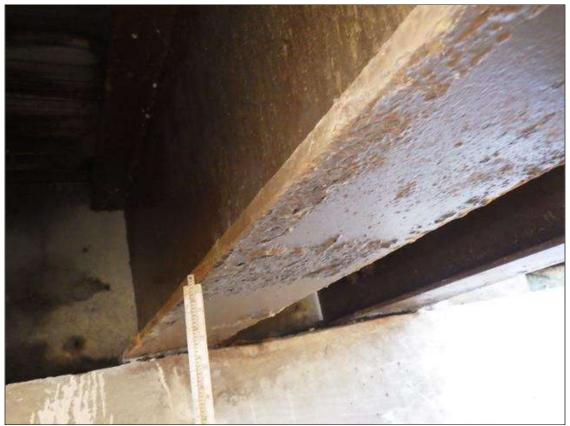
Span 1 Beam 2: ARRESTED CORROSION UP TO 4 FEET 6 INCHES LONG X FULL WIDTH WITH 1/32 INCH SECTION LOSS IN THE BOTTOM FLANGE AT END BENT 1
