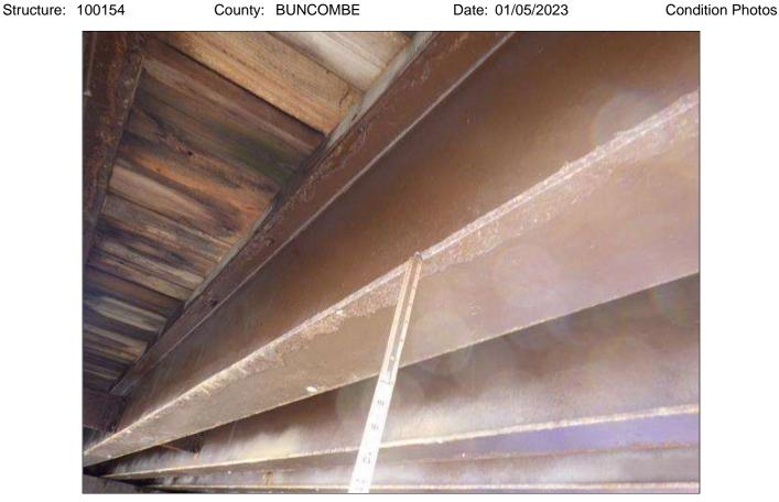
Span 1 Beam 8: ARRESTED CORROSION UP TO INTERMITTENT FULL LENGTH X INTERMITTENT FULL WIDTH WITH 1/32 INCH SECTION LOSS IN THE BOTTOM FLANGE
