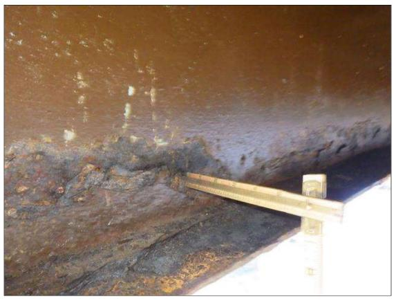
Span 2 Beam 9: ARRESTED CORROSION UP TO 7 FEET 8 INCHES LONG X 8 INCHES HIGH WITH 5/16 INCH REMAINING (GREATER THAN OR EQUAL TO 1/16 INCH SECTION LOSS, LESS THAN 25 PERCENT SECTION LOSS) IN THE WEB AT END BENT 2
