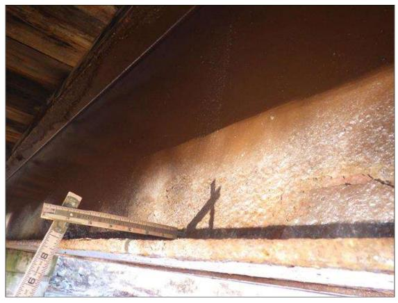
Span 2 Beam 5: ARRESTED CORROSION UP TO FULL LENGTH X 6 INCHES HIGH WITH 5/16 INCH REMAINING (GREATER THAN OR EQUAL TO 1/16 INCH SECTION LOSS, LESS THAN 25 PERCENT SECTION LOSS) IN THE WEB
