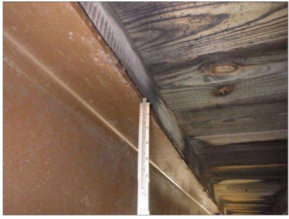
Span 1 Beam 2: ARRESTED CORROSION UP TO FULL LENGTH X 1 INCH WIDE WITH 1/32 INCH SECTION LOSS IN THE TOP FLANGE EDGES
