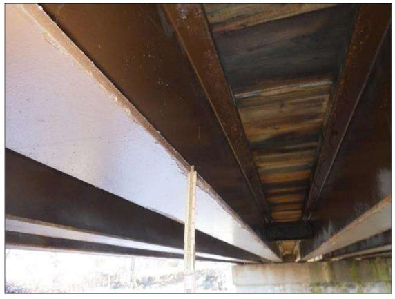
Span 2 Beam 7: ARRESTED CORROSION UP TO INTERMITTENT FULL LENGTH X FULL WIDTH WITH 1/32 INCH SECTION LOSS IN THE BOTTOM FLANGE
