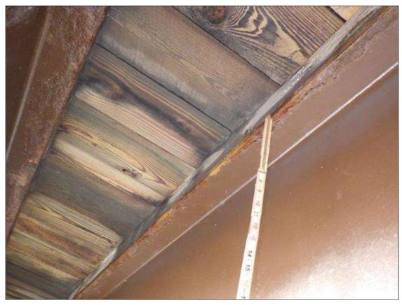
Span 1 Beam 7: ARRESTED CORROSION UP TO FULL LENGTH X FULL WIDTH WITH 7/16 INCH REMAINING (GREATER THAN OR EQUAL TO 1/16 INCH SECTION LOSS, LESS THAN 25 PERCENT SECTION LOSS) IN THE TOP FLANGE
