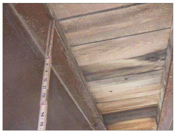
Span 1 Beam 8: ARRESTED CORROSION UP TO FULL LENGTH X FULL WIDTH WITH 7/16 INCH REMAINING (GREATER THAN OR EQUAL TO 1/16 INCH SECTION LOSS, LESS THAN 25 PERCENT SECTION LOSS) IN THE TOP FLANGE
