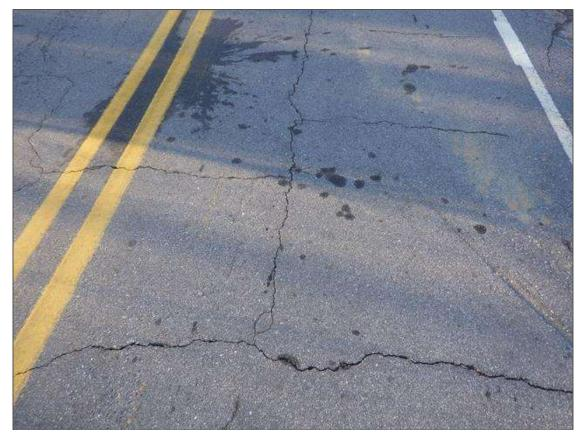
MAP CRACKING UP TO INTERMITTENT FULL WIDTH X GREATER THAN 150 FEET LONG X 1/8 INCH WIDE IN THE SOUTH APPROACH AT END BENT 1
