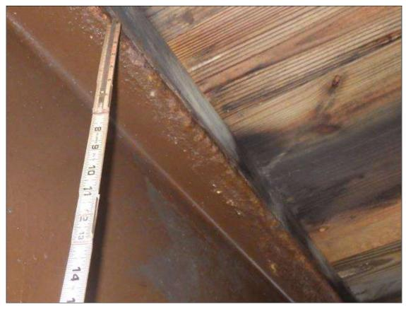
Span 2 Beam 3: ARRESTED CORROSION UP TO INTERMITTENT FULL LENGTH X FULL WIDTH WITH 7/16 INCH REMAINING (GREATER THAN OR EQUAL TO 1/16 INCH SECTION LOSS, LESS THAN 25 PERCENT SECTION LOSS) IN THE TOP FLANGE
