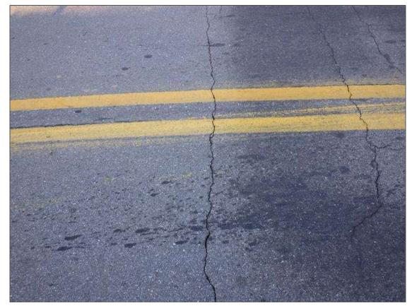
Span 1 Wearing Surface: TRANSVERSE CRACK UP TO FULL WIDTH X 1/4 INCH WIDE AT END BENT 1
