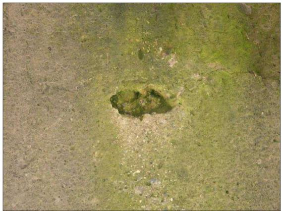
Bent 1 Cap 1: SPALLED AREA UP TO 3 INCHES LONG X 2 INCHES HIGH X 1 INCH DEEP IN THE NORTH FACE BELOW BEAM 4
