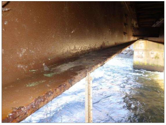
Span 1 Beam 1: ARRESTED CORROSION UP TO INTERMITTENT FULL LENGTH X FULL WIDTH WITH 1/32 INCH SECTION LOSS IN THE BOTTOM FLANGE
