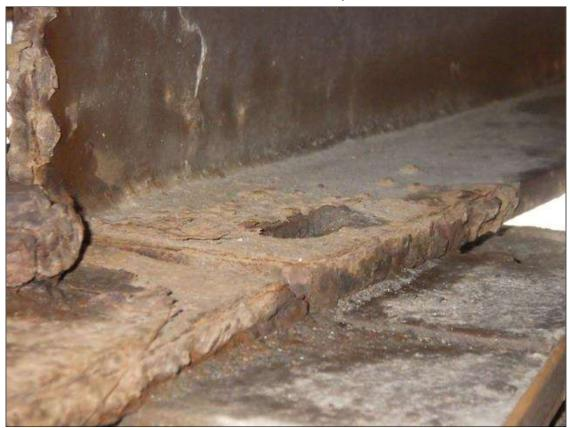
Span 1 Near Bearing: MISSING LEFT ANCHOR BOLT IN BEAM 5 BEARING (PRIORITY ACTION REQUEST)
