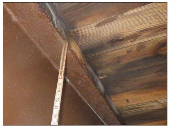
Span 2 Beam 2: ARRESTED CORROSION UP TO INTERMITTENT FULL LENGTH X FULL WIDTH WITH 7/16 INCH REMAINING (GREATER THAN OR EQUAL TO 1/16 INCH SECTION LOSS, LESS THAN 25 PERCENT SECTION LOSS) IN THE TOP FLANGE
