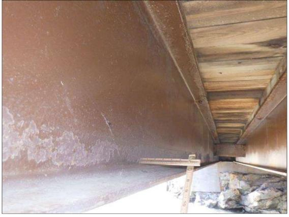
Span 1 Beam 8: ARRESTED CORROSION UP TO INTERMITTENT FULL LENGTH X 8 INCHES HIGH WITH 1/32 INCH SECTION LOSS IN THE WEB
