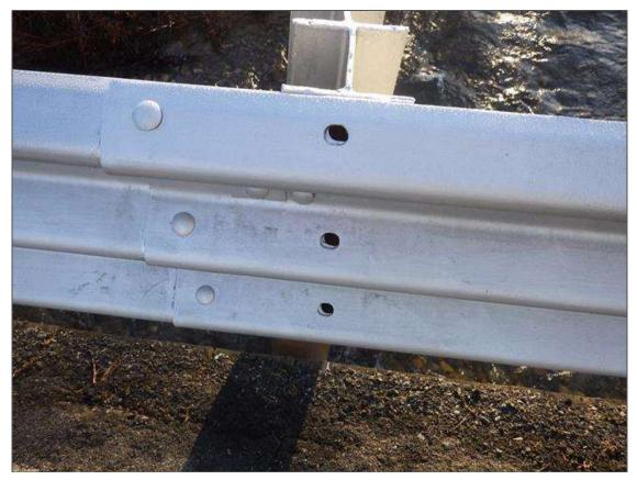
Span 1 Right Bridge Rail: MISSING (3) ANCHOR BOLTS AT POST 5 (PRIORITY ACTION REQUEST)
