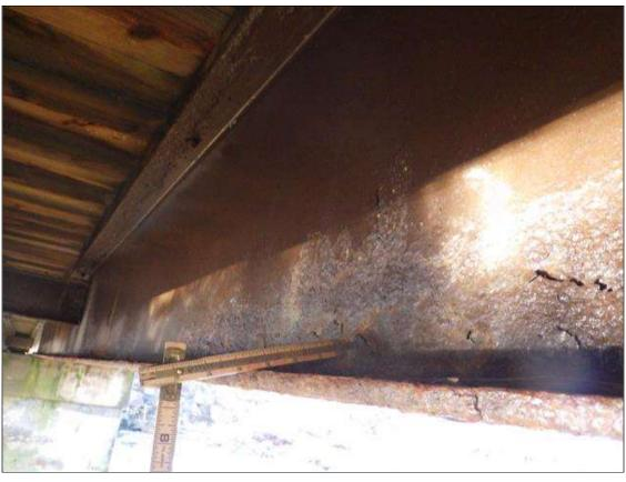
Span 2 Beam 3: ARRESTED CORROSION UP TO INTERMITTENT FULL LENGTH X INTERMITTENT FULL HEIGHT WITH 5/16 INCH REMAINING (GREATER THAN OR EQUAL TO 1/16 INCH SECTION LOSS, LESS THAN 25 PERCENT SECTION LOSS) IN THE WEB
