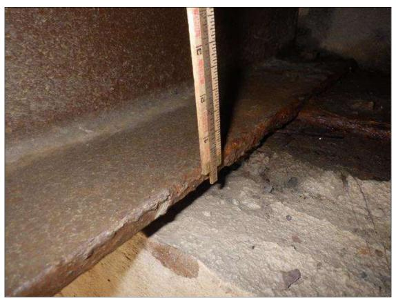
Span 1 Beam 5: ARRESTED CORROSION UP TO 1 FOOT 6 INCHES LONG X FULL WIDTH WITH 1/32 INCH SECTION LOSS IN THE BOTTOM FLANGE AT END BENT 1
