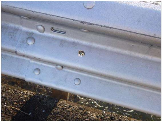
Span 1 Right Bridge Rail: MISSING (1) ANCHOR BOLT AT POST 3 (PRIORITY ACTION REQUEST)
