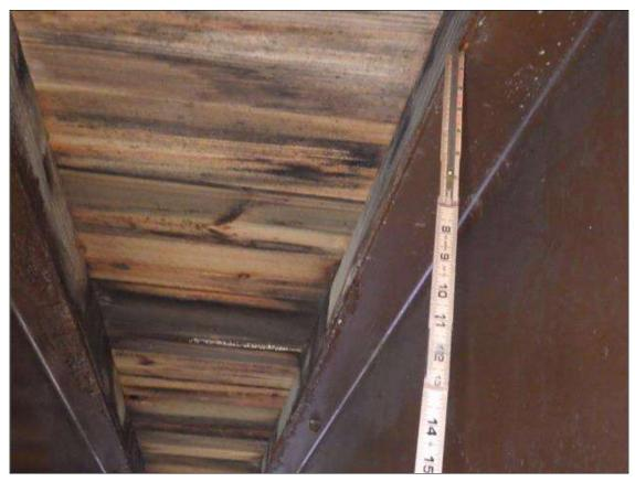
Span 2 Beam 7: ARRESTED CORROSION UP TO INTERMITTENT FULL LENGTH X FULL WIDTH WITH 7/16 INCH REMAINING (GREATER THAN OR EQUAL TO 1/16 INCH SECTION LOSS, LESS THAN 25 PERCENT SECTION LOSS) IN THE TOP FLANGE
