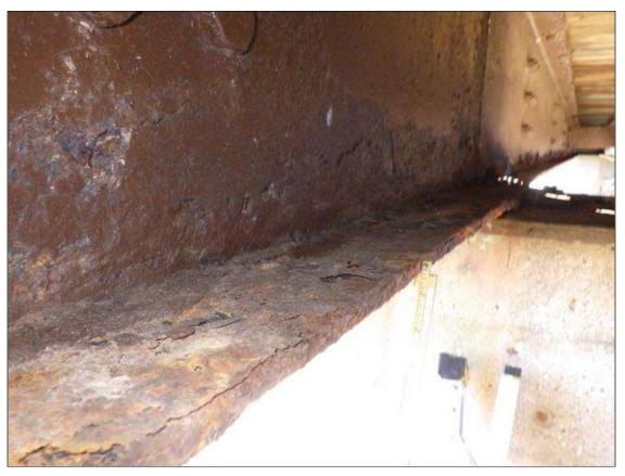
Span 2 Beam 9: ARRESTED CORROSION UP TO 16 FEET 9 INCHES LONG X FULL WIDTH WITH 3/8 INCH REMAINING (GREATER THAN OR EQUAL TO 1/16 INCH SECTION LOSS, GREATER THAN 25 PERCENT SECTION LOSS) IN THE BOTTOM FLANGE AT BENT 1 (PRIORITY ACTION REQUEST)
