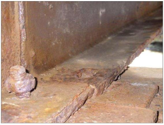
Span 1 Near Bearing: MISSING LEFT ANCHOR BOLT IN BEAM 2 BEARING (PRIORITY ACTION REQUEST)
