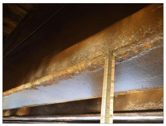
Span 2 Beam 5: ARRESTED CORROSION UP TO INTERMITTENT FULL LENGTH X INTERMITTENT FULL WIDTH WITH 7/16 INCH REMAINING (GREATER THAN OR EQUAL TO 1/16 INCH SECTION LOSS, LESS THAN 25 PERCENT SECTION LOSS) IN THE BOTTOM FLANGE
