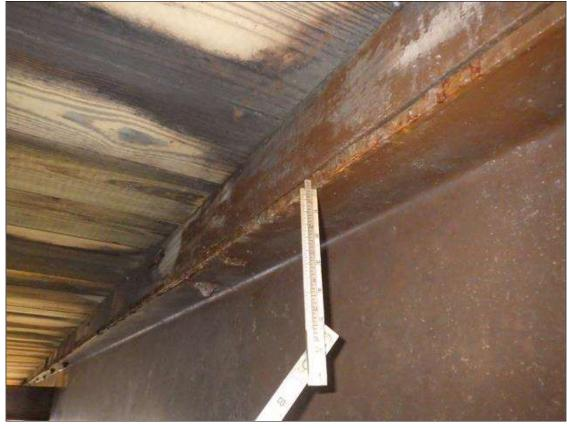
Span 1 Beam 4: ARRESTED CORROSION UP TO INTERMITTENT FULL LENGTH X FULL WIDTH WITH 1/32 INCH SECTION LOSS IN THE TOP FLANGE
