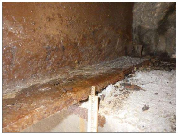
Span 2 Beam 8: ARRESTED CORROSION UP TO 1 FOOT 6 INCHES LONG X FULL WIDTH WITH 7/16 INCH REMAINING (GREATER THAN OR EQUAL TO 1/16 INCH SECTION LOSS, LESS THAN 25 PERCENT SECTION LOSS) IN THE BOTTOM FLANGE AT END BENT 2
