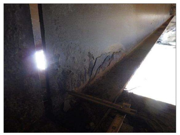
Span 1 Beam 6: CORROSION UP TO 1 FOOT 10 INCHES LONG X 8 INCHES HIGH WITH 1/32 INCH SECTION LOSS IN THE WEB AT BENT 1
