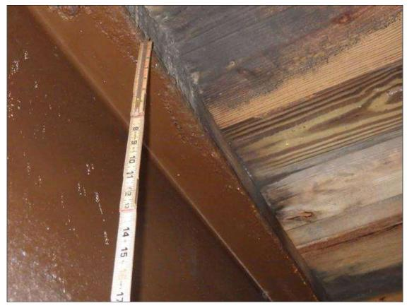
Span 2 Beam 5: ARRESTED CORROSION UP TO INTERMITTENT FULL LENGTH X FULL WIDTH WITH 7/16 INCH REMAINING (GREATER THAN OR EQUAL TO 1/16 INCH SECTION LOSS, LESS THAN 25 PERCENT SECTION LOSS) IN THE TOP FLANGE
