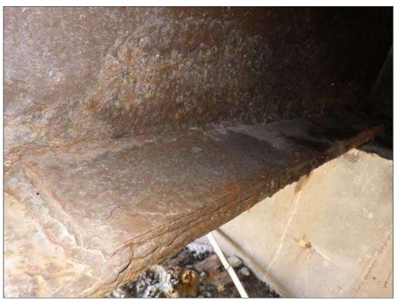
Span 1 Beam 7: (2) REPAIR PLATES UP TO 2 FEET 6 INCHES LONG X 3 1/2 INCHES WIDE X 1/2 INCH THICK IN THE BOTTOM LEFT FLANGE AND 3 FEET 4 INCHES LONG X 3 1/2 INCHES WIDE X 1/2 INCH THICK IN THE BOTTOM RIGHT FLANGE AT END BENT 1
