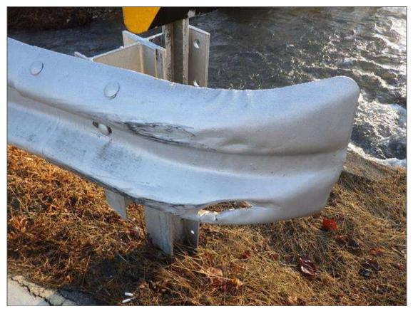
Span 1 Right Bridge Rail: IMPACT DAMAGE UP TO 2 FEET LONG WITH HOLE UP TO 3 INCHES LONG X 1 INCH HIGH IN THE SOUTH END TERMINAL (PRIORITY ACTION REQUEST)
