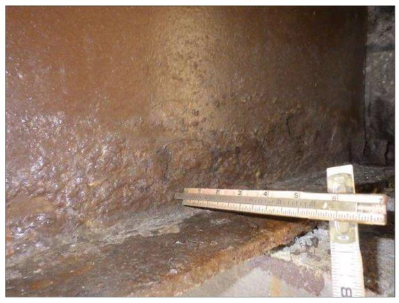
Span 2 Beam 8: ARRESTED CORROSION UP TO 1 FOOT 6 INCHES LONG X 4 INCHES HIGH WITH 5/16 INCH REMAINING (GREATER THAN OR EQUAL TO 1/16 INCH SECTION LOSS, LESS THAN 25 PERCENT SECTION LOSS) IN THE WEB AT END BENT 2
