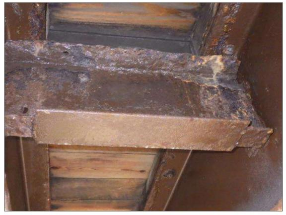
Span 2 Beam 6: REPAIR ANGLE UP TO 1 FOOT LONG X 4 INCHES WIDE X 4 INCHES HIGH IN BAY 6 INTERMEDIATE DIAPHRAGM
