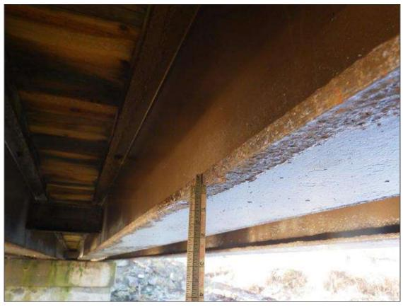
Span 2 Beam 2: ARRESTED CORROSION UP TO INTERMITTENT FULL LENGTH X FULL WIDTH WITH 1/32 INCH SECTION LOSS IN THE BOTTOM FLANGE
