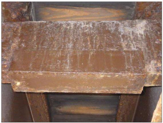
Span 2 Beam 2: REPAIR ANGLE UP TO 1 FOOT LONG X 4 INCHES WIDE X 4 INCHES HIGH IN BAY 2 INTERMEDIATE DIAPHRAGM
