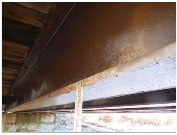
Span 2 Beam 6: ARRESTED CORROSION UP TO FULL LENGTH X INTERMITTENT FULL WIDTH WITH 7/16 INCH REMAINING (GREATER THAN OR EQUAL TO 1/16 INCH SECTION LOSS, LESS THAN 25 PERCENT SECTION LOSS) IN THE BOTTOM FLANGE
