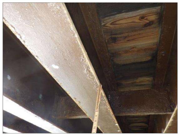
Span 1 Beam 6: ARRESTED CORROSION UP TO INTERMITTENT FULL LENGTH X INTERMITTENT FULL WIDTH WITH 1/32 INCH SECTION LOSS IN THE BOTTOM FLANGE
