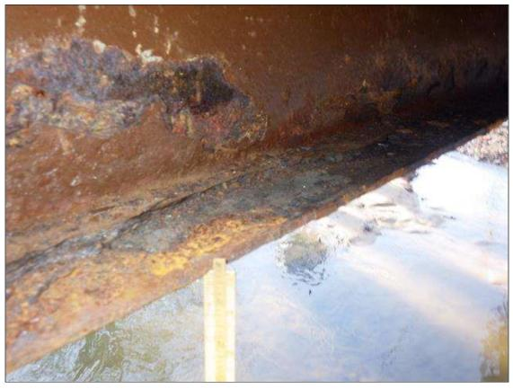
Span 2 Beam 9: ACTIVE CORROSION UP TO 7 FEET 8 INCHES LONG X FULL WIDTH WITH 3/16 INCH REMAINING (GREATER THAN OR EQUAL TO 1/16 INCH SECTION LOSS, GREATER THAN 25 PERCENT SECTION LOSS) IN THE BOTTOM FLANGE AT END BENT 2 (PRIORITY ACTION REQUEST)
