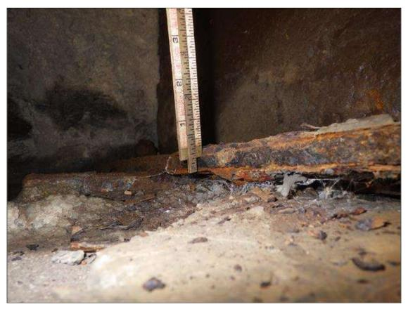
Span 1 Beam 3: ACTIVE CORROSION UP TO 1 FOOT 4 INCHES LONG X FULL WIDTH WITH 3/8 INCH REMAINING (GREATER THAN OR EQUAL TO 1/16 INCH SECTION LOSS, GREATER THAN 25 PERCENT SECTION LOSS) IN THE BOTTOM FLANGE AT END BENT 1 (PRIORITY ACTION REQUEST)
