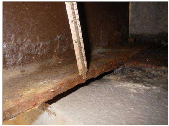
Span 1 Beam 4: ARRESTED CORROSION UP TO 2 FEET LONG X FULL WIDTH WITH 1/32 INCH SECTION LOSS IN THE BOTTOM FLANGE AT END BENT 1
