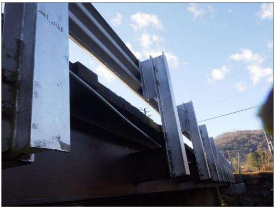
(1) 3/4 INCH DIAMETER POLYVINYL CHLORIDE CONDUIT UTILITY ALONG THE WEST OVERHANG
