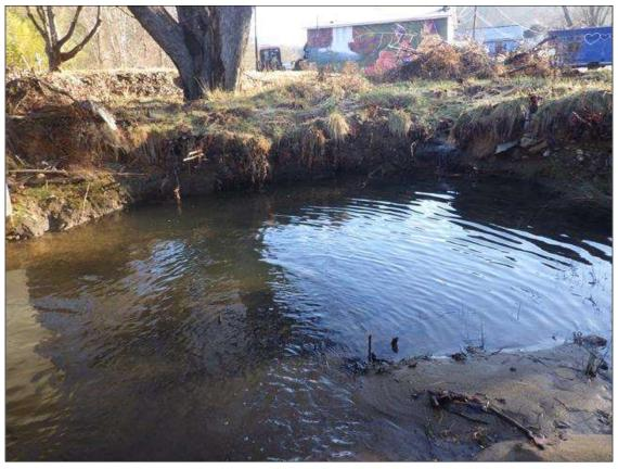
SCOUR HOLE UP TO 20 FEET DIAMETER X 3 FEET DEEP AT THE EAST END OF END BENT 2
