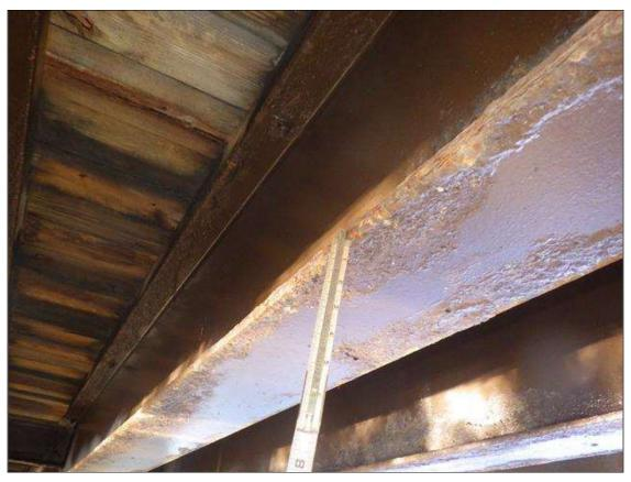
Span 2 Beam 4: ARRESTED CORROSION UP TO FULL LENGTH X FULL WIDTH WITH 7/16 INCH REMAINING (GREATER THAN OR EQUAL TO 1/16 INCH SECTION LOSS, LESS THAN 25 PERCENT SECTION LOSS) IN THE BOTTOM FLANGE
