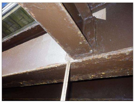
Span 1 Beam 9: ARRESTED CORROSION UP TO INTERMITTENT FULL LENGTH X FULL WIDTH WITH 7/16 INCH REMAINING (GREATER THAN OR EQUAL TO 1/16 INCH SECTION LOSS, LESS THAN 25 PERCENT SECTION LOSS) IN THE BOTTOM FLANGE
