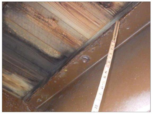
Span 1 Beam 5: ARRESTED CORROSION UP TO INTERMITTENT FULL LENGTH X 1 INCH WIDE WITH 7/16 INCH REMAINING (GREATER THAN OR EQUAL TO 1/16 INCH SECTION LOSS, LESS THAN 25 PERCENT SECTION LOSS) IN THE TOP FLANGE EDGES
