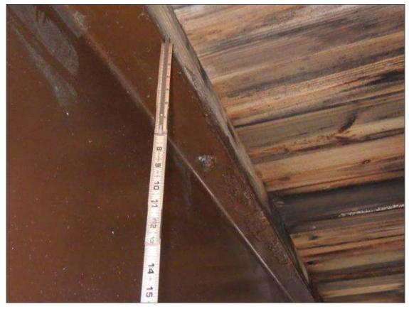
Span 2 Beam 8: ARRESTED CORROSION UP TO INTERMITTENT FULL LENGTH X FULL WIDTH WITH 7/16 INCH REMAINING (GREATER THAN OR EQUAL TO 1/16 INCH SECTION LOSS, LESS THAN 25 PERCENT SECTION LOSS) IN THE TOP FLANGE
