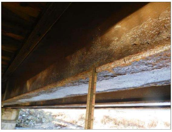
Span 2 Beam 3: ARRESTED CORROSION UP TO INTERMITTENT FULL LENGTH X FULL WIDTH WITH 7/16 INCH REMAINING (GREATER THAN OR EQUAL TO 1/16 INCH SECTION LOSS, LESS THAN 25 PERCENT SECTION LOSS) IN THE BOTTOM FLANGE
