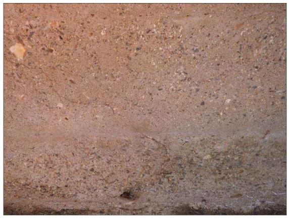
Bent 1 Pile 1: MAP CRACKING UP TO FULL LENGTH X FULL HEIGHT X 1/32 INCH WIDE IN THE NORTH AND SOUTH FACES
