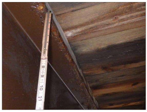
Span 2 Beam 4: ARRESTED CORROSION UP TO INTERMITTENT FULL LENGTH X FULL WIDTH WITH 7/16 INCH REMAINING (GREATER THAN OR EQUAL TO 1/16 INCH SECTION LOSS, LESS THAN 25 PERCENT SECTION LOSS) IN THE TOP FLANGE
