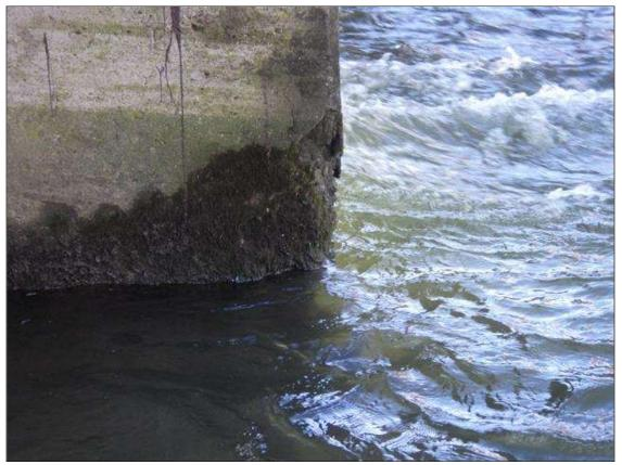
Bent 1 Pile 1: SPALLED AREA UP TO 6 INCHES LONG X 2 FEET WIDE X 4 FEET HIGH WITH EXPOSED REINFORCEMENT IN THE NORTHWEST CORNER, 4 FEET BELOW CAP
