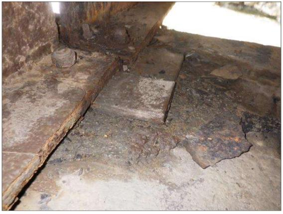
BEAM 6 BEARING AT BENT 1 REPAINTED PRIOR TO 2023 INSPECTION CYCLE (OTHERS SIMILAR)
