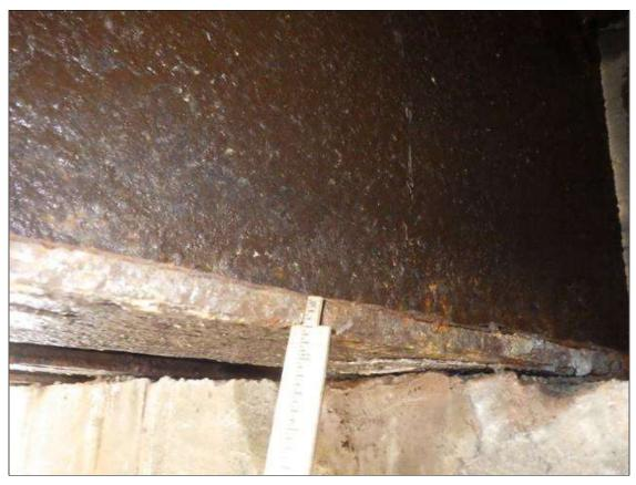
Span 1 Beam 6: ARRESTED CORROSION UP TO 3 FEET 4 INCHES LONG X FULL WIDTH WITH 7/16 INCH REMAINING (GREATER THAN OR EQUAL TO 1/16 INCH SECTION LOSS, LESS THAN 25 PERCENT SECTION LOSS) IN THE BOTTOM FLANGE AT END BENT 1
