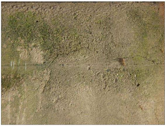
Bent 1 Cap 1: MAP CRACKING UP TO INTERMITTENT FULL LENGTH X FULL WIDTH X FULL HEIGHT X 1/32 INCH WIDE IN THE NORTH AND SOUTH FACES
