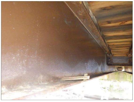
Span 2 Beam 4: ARRESTED CORROSION UP TO INTERMITTENT FULL LENGTH X 8 INCHES HIGH WITH 5/16 INCH REMAINING (GREATER THAN OR EQUAL TO 1/16 INCH SECTION LOSS, LESS THAN 25 PERCENT SECTION LOSS) IN THE WEB
