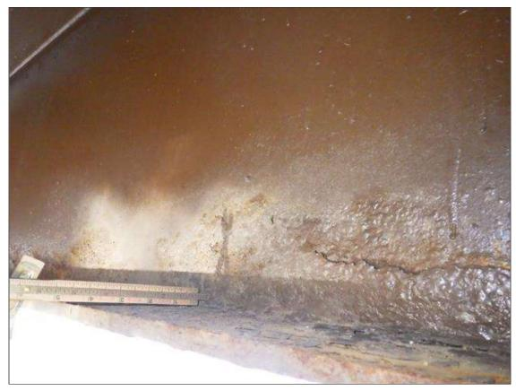
Span 2 Beam 6: ARRESTED CORROSION UP TO INTERMITTENT FULL LENGTH X 6 INCHES HIGH WITH 5/16 INCH REMAINING (GREATER THAN OR EQUAL TO 1/16 INCH SECTION LOSS, LESS THAN 25 PERCENT SECTION LOSS) IN THE WEB
