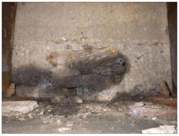
End Bent 2 Abutment: SPALLED AREA UP TO 9 INCHES LONG X 6 INCHES HIGH X 2 INCHES DEEP BELOW BAY 6 IN THE BACKWALL
