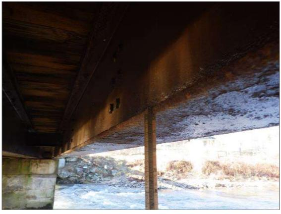
Span 2 Beam 1: ARRESTED CORROSION UP TO FULL LENGTH X FULL WIDTH WITH 7/16 INCH REMAINING (GREATER THAN OR EQUAL TO 1/16 INCH SECTION LOSS, LESS THAN 25 PERCENT SECTION LOSS) IN THE BOTTOM FLANGE
