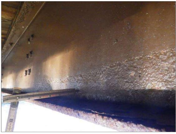
Span 2 Beam 1: ARRESTED CORROSION UP TO INTERMITTENT FULL LENGTH X 6 INCHES HIGH WITH 1/32 INCH SECTION LOSS IN THE WEB
