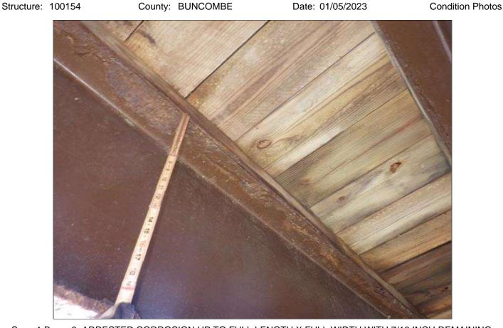
Span 1 Beam 9: ARRESTED CORROSION UP TO FULL LENGTH X FULL WIDTH WITH 7/16 INCH REMAINING (GREATER THAN OR EQUAL TO 1/16 INCH SECTION LOSS, LESS THAN 25 PERCENT SECTION LOSS) IN THE TOP FLANGE
