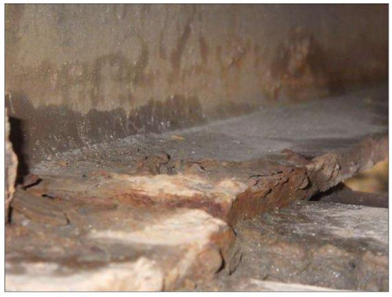
Span 1 Near Bearing: MISSING LEFT ANCHOR BOLT AND ANCHOR BOLT NUT IN BEAM 4 BEARING (PRIORITY ACTION REQUEST)
