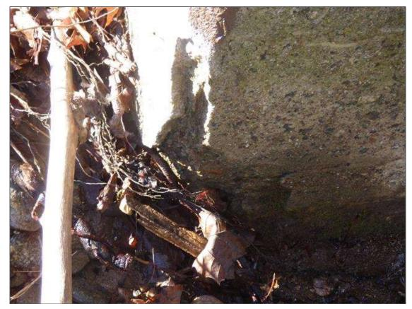
Bent 1 Pile 1: SPALLED AREA UP TO 6 INCHES LONG X 5 INCHES WIDE X 1 FOOT HIGH IN THE NORTHEAST CORNER, 3 FEET BELOW CAP
