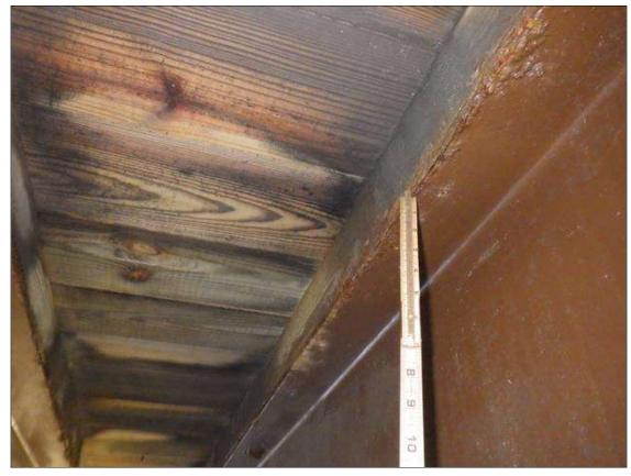
Span 1 Beam 3: ARRESTED CORROSION UP TO INTERMITTENT FULL LENGTH X FULL WIDTH WITH 1/32 INCH SECTION LOSS IN THE TOP FLANGE
