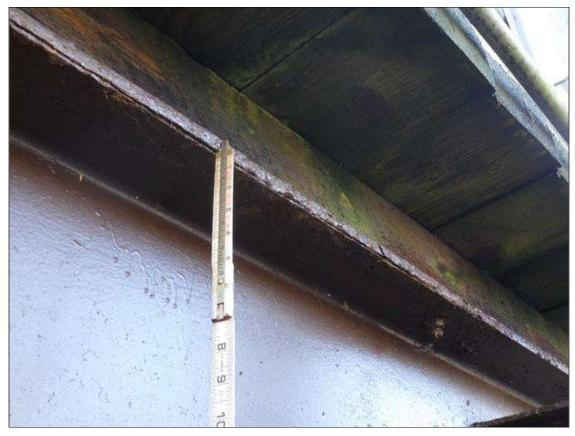
Span 2 Beam 1: ARRESTED CORROSION UP TO INTERMITTENT FULL LENGTH X FULL WIDTH WITH 7/16 INCH REMAINING (GREATER THAN OR EQUAL TO 1/16 INCH SECTION LOSS, LESS THAN 25 PERCENT SECTION LOSS) IN THE TOP FLANGE
