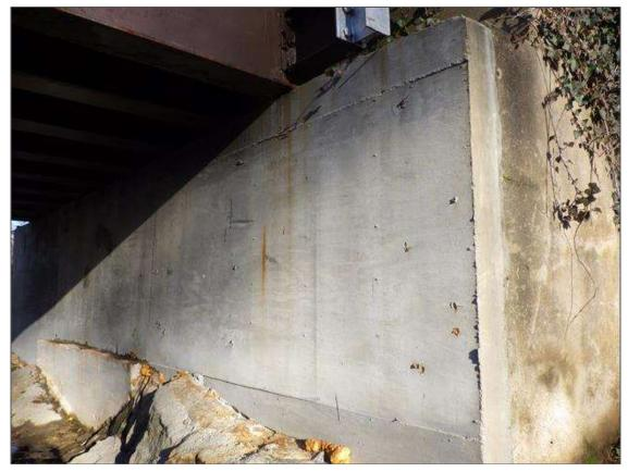
End Bent 2 Abutment: REPAIR PATCH AREA UP TO FULL LENGTH X 6 FEET HIGH X 6 INCHES THICK
