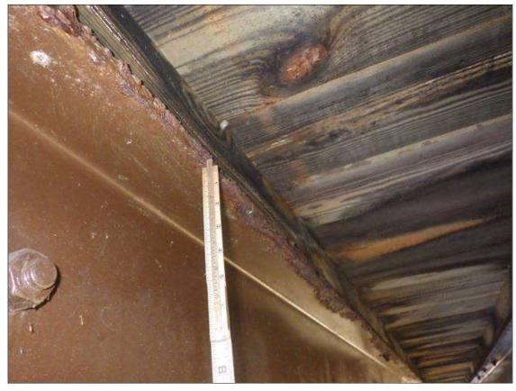
Span 1 Beam 1: ARRESTED CORROSION UP TO FULL LENGTH X FULL HEIGHT WITH 5/16 INCH REMAINING (GREATER THAN OR EQUAL TO 1/16 INCH SECTION LOSS, LESS THAN 25 PERCENT SECTION LOSS) IN THE WEB
