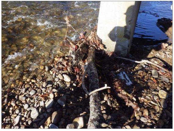
DRIFT UP TO 2 FEET DIAMETER X 30 FEET LONG AT THE UPSTREAM END OF BENT 1
